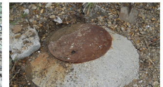
A non-corroded manhole on land.
